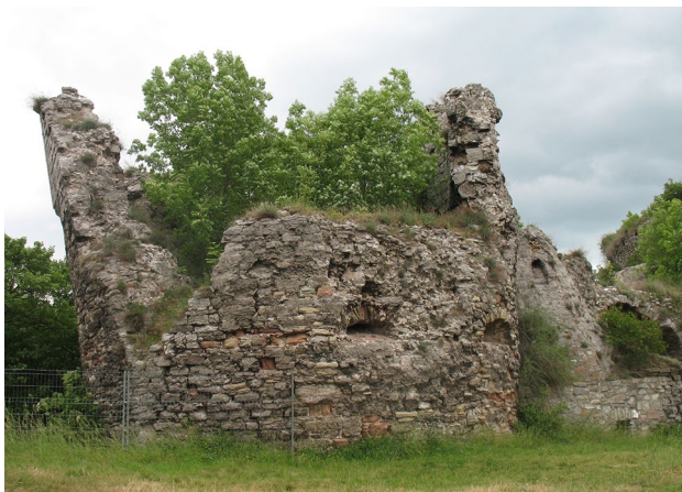
Fig. 6 Ruined tower of the Wendelstein castle (Memleben). Volume expansion of building stones upon uptake of water of the anhydrite causes inclination or bending of walls, but also refilling of existing clefts
