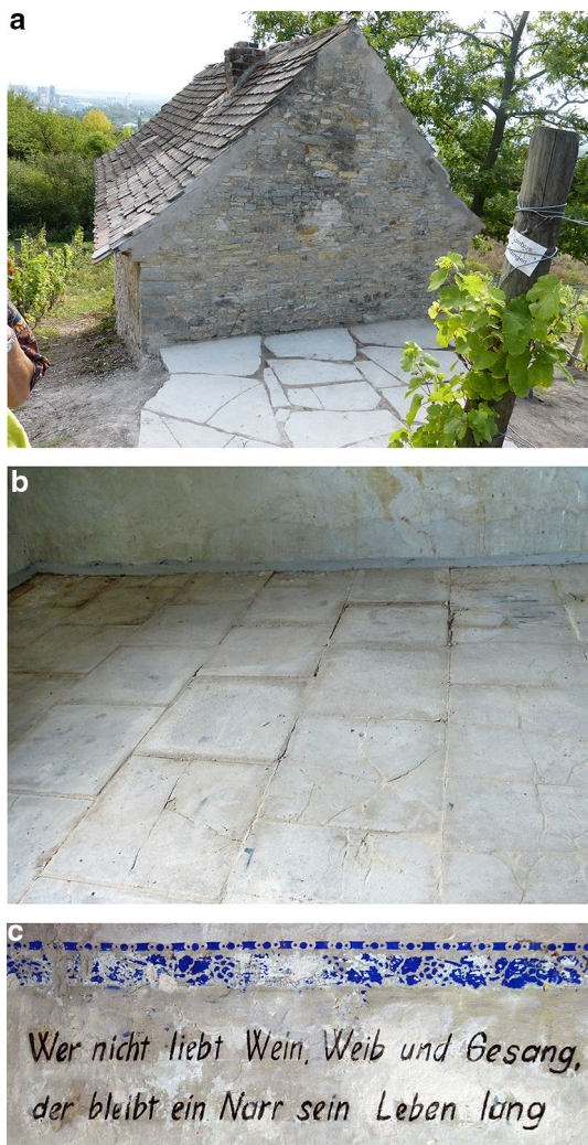
Fig. 10 Kathert's vineyard cabin after restoration. a Behind the cabin, limestone tiles for a small terrace were laid. b Restored floor tiles of the central room. c Wall section with banner
